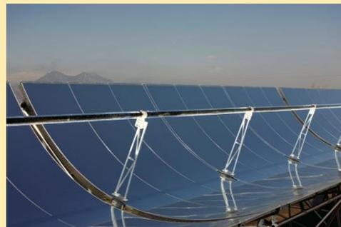
Figure 1: Parabolic Trough plant [1]
