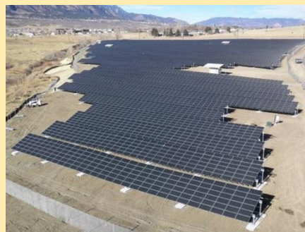
Figure 1: Photovoltaic power plant [1]
